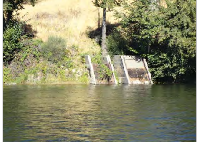
PHOTO 3: Abandoned concrete pads on the north bank of the American River.
